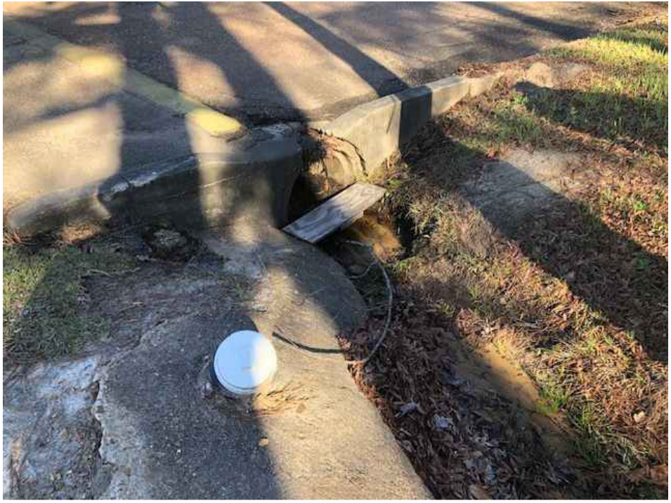
8 24" PIPE ON EAST SIDE OF EMERALD DR.
