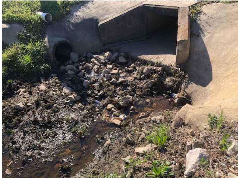
1 LOOKING SOUTH BOX CULVERT UNDER HWY 182
