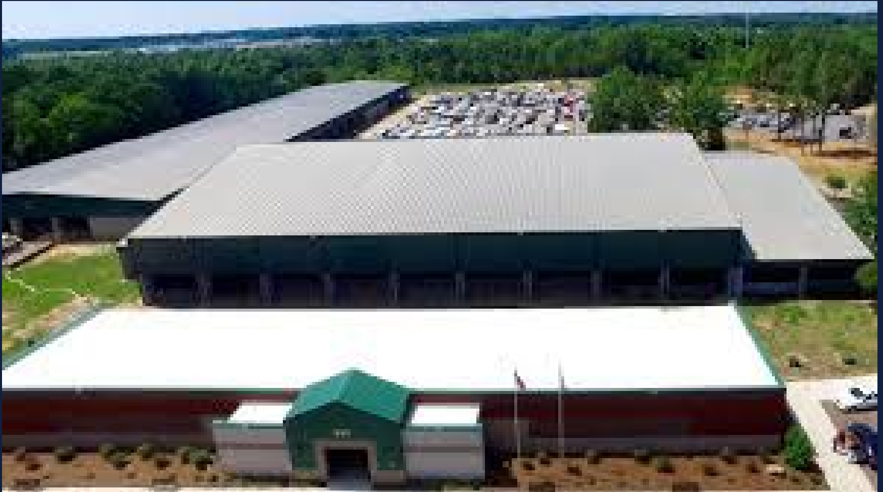
Rankin County Safe Room
