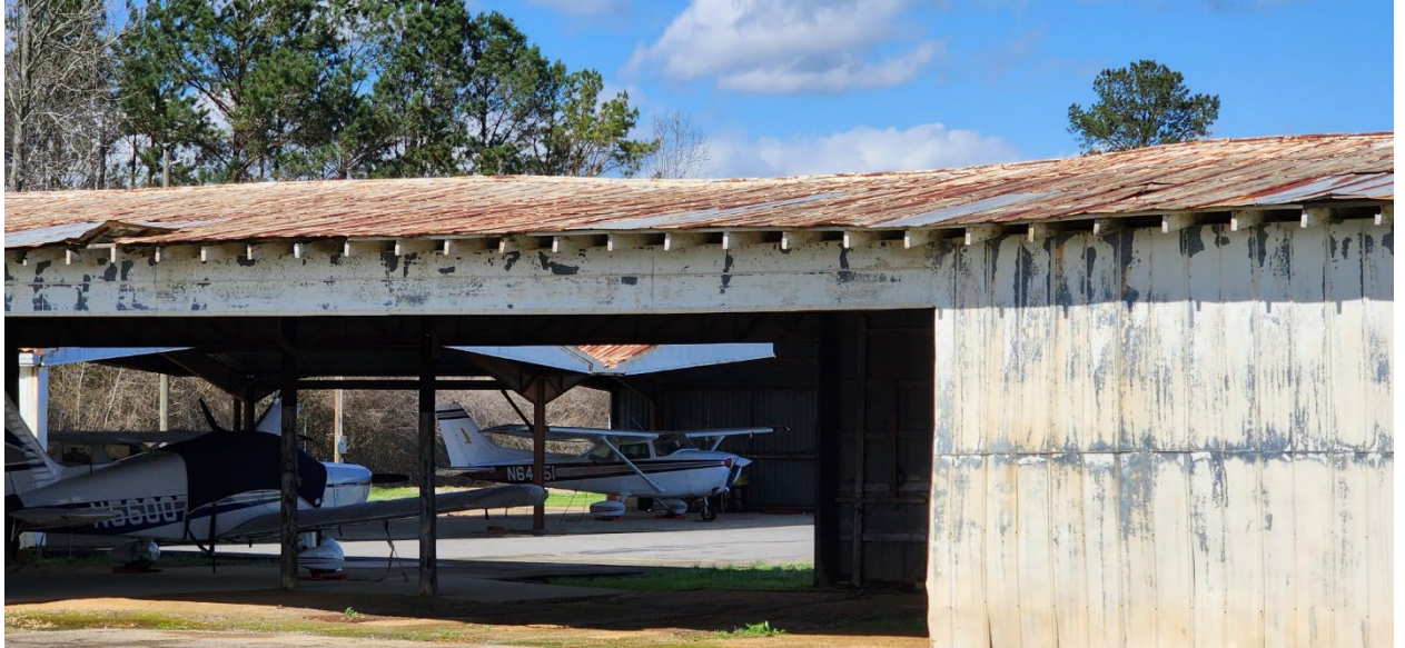
Photo 3 – South Side of Hangar
