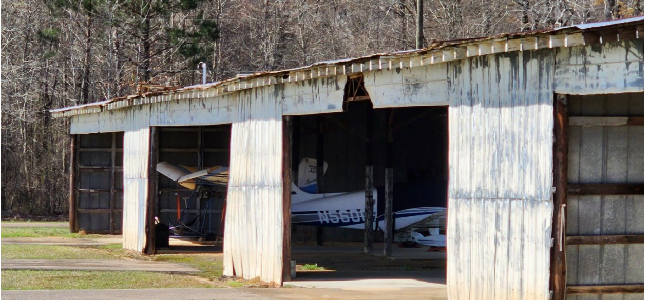
Photo 1 – South Side of Existing Hangar
