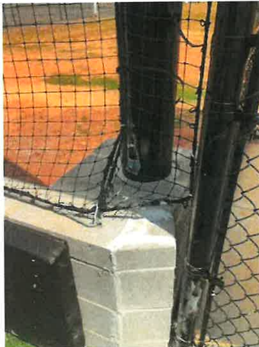
Photo 6 – Re-Attach All Pads, Typical All Fields.
