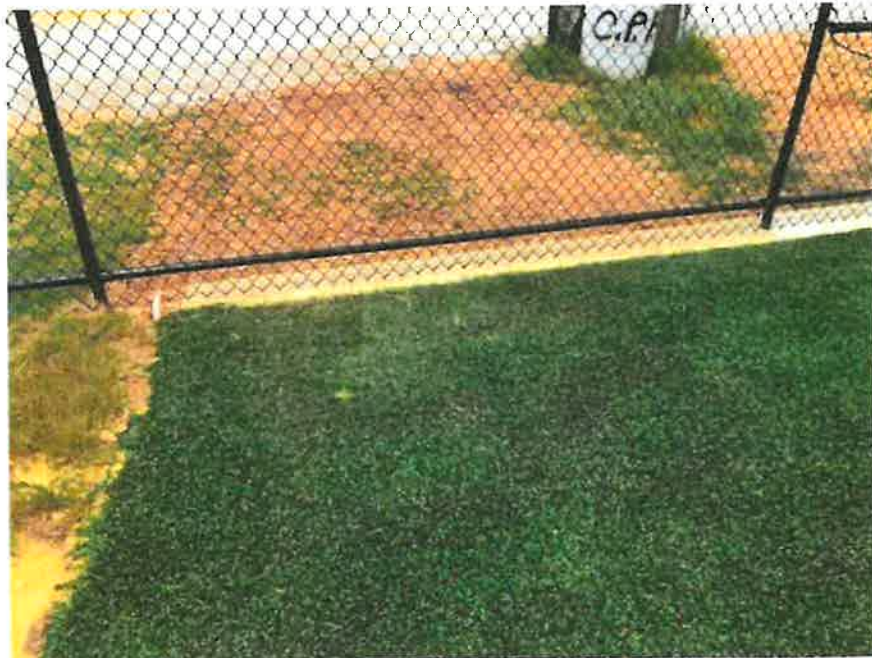
Photo 2 – Lower Fence Bottom Rails To Prevent Balls From Escaping.
