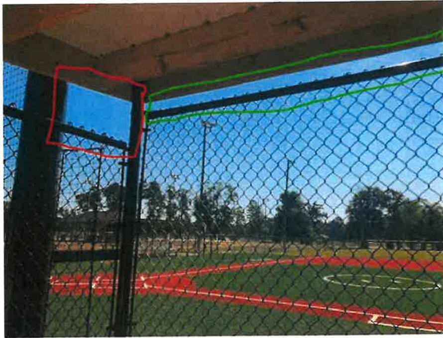
Photo 11 – Extend Corner Netting To Top of Dugout Roofline, Typical All.
