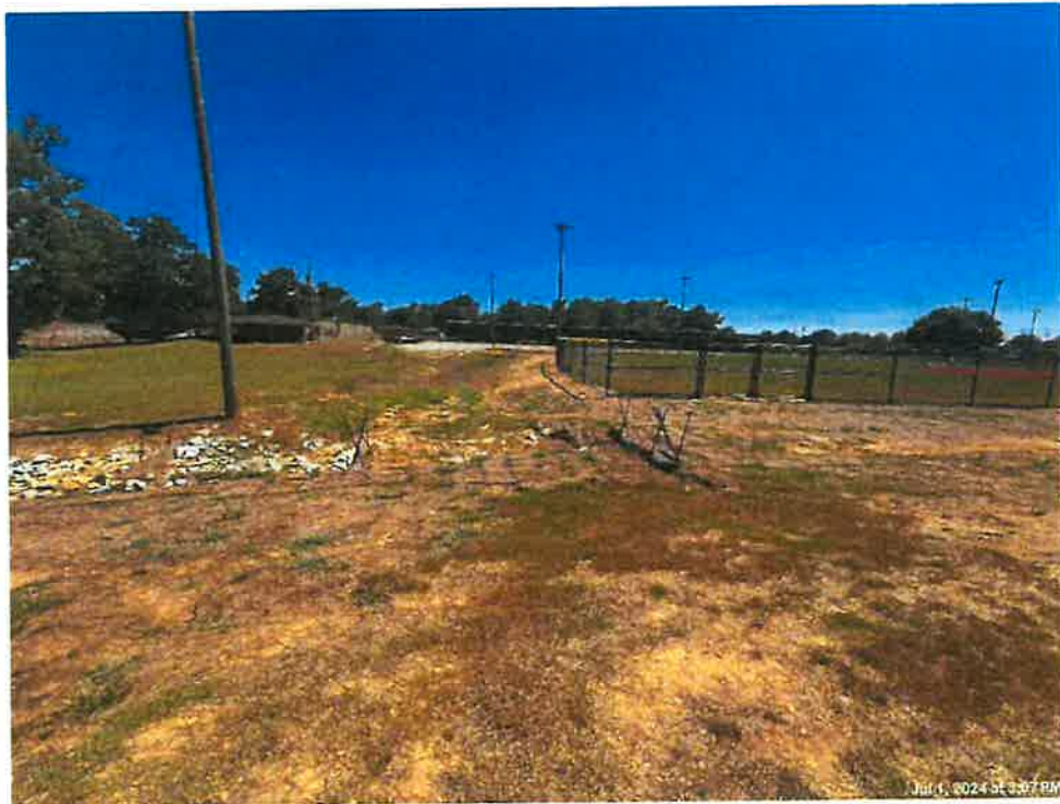
Photo 10 – Re-Seed and Hay Areas Not Disturbed By The Field Lighting and Concrete Package.
