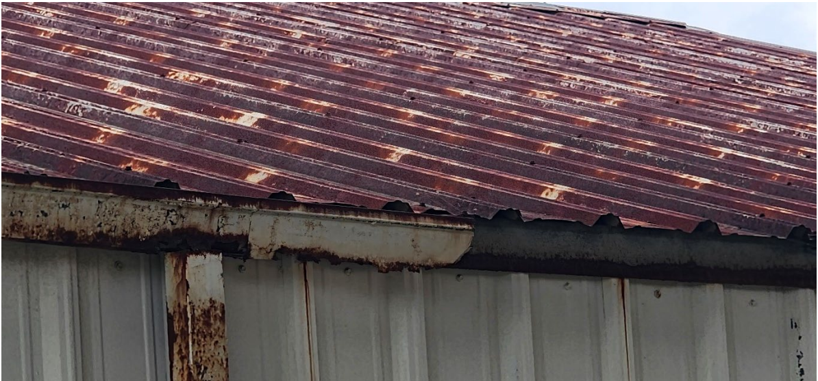
Photo 2 – Roof/Downspout Corrosion
