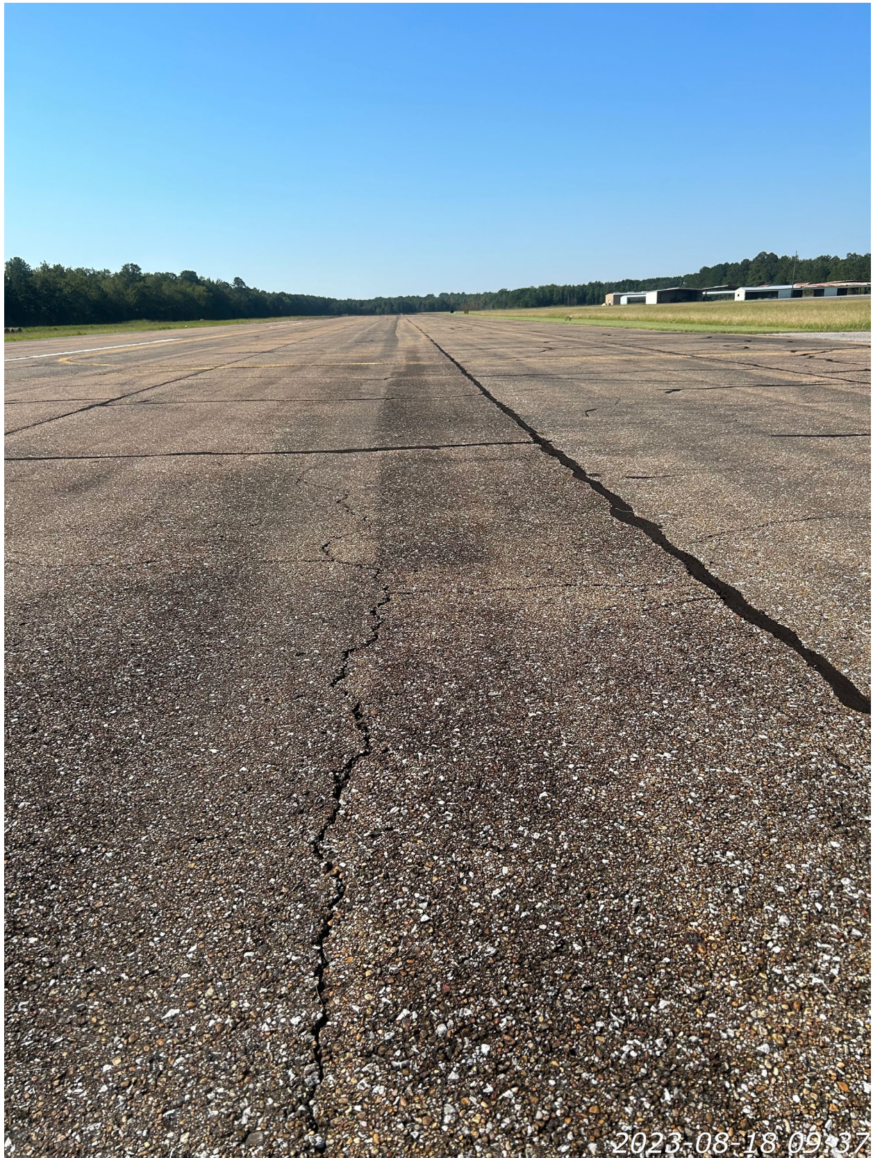
Photo 6 – Block Cracking and Oxidation in Runway Pavement
