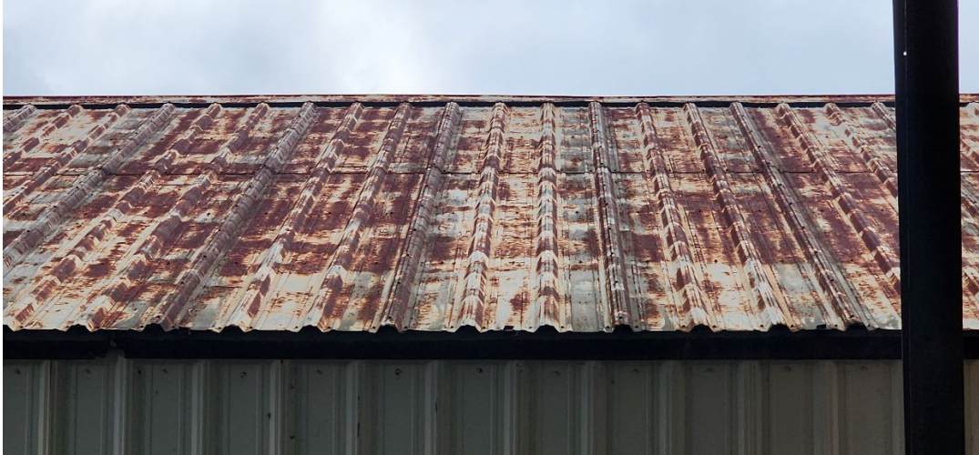
Photo 3 – Roof Corrosion
