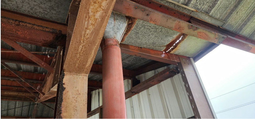
Photo 6 – Gutter Leak
