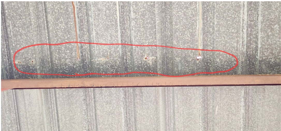
Photo 4 – Roof Leaks
