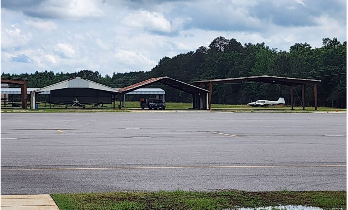
Photo 1 – North Side of Hangars to be Rehabilitated
