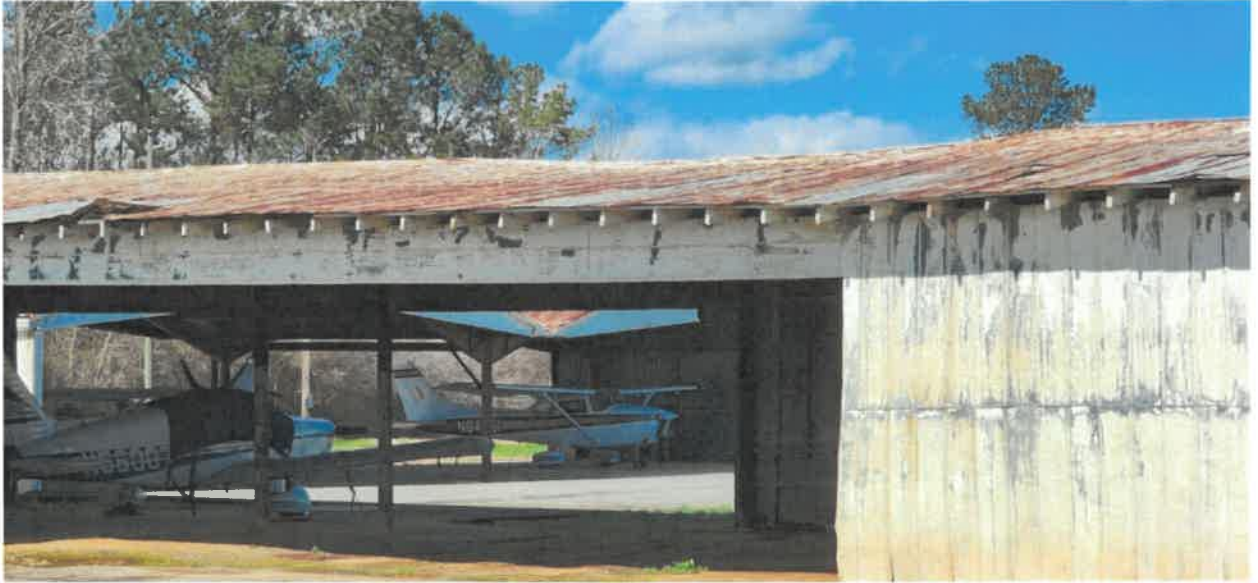
Photo 3 – South Side of Hangar
