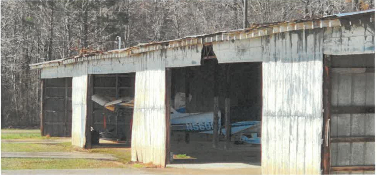
Photo 1 – South Side of Existing Hangar
