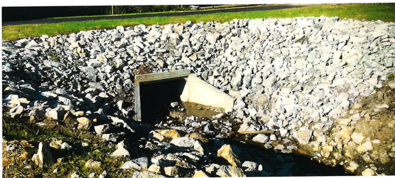
2nd Avenue Culvert Replacement, Columbus, MS
