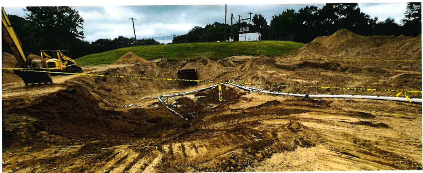
22nd Street South Lift Station Renovation
