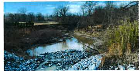
Accelerated rain events have meant more erosion that has widened the Paces Bayou drainage channel to 200 feet in some places. Neel-Schaffer has designed a solution to restore and stabilize the bank that includes 14,000 tons of riprap rock.
