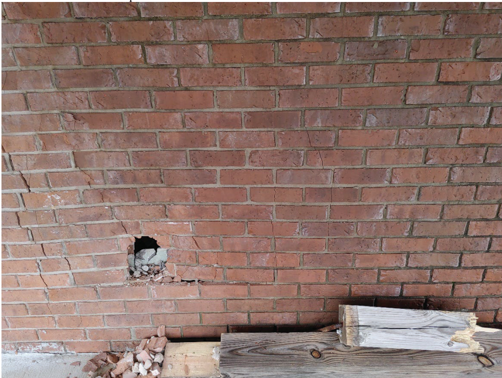
6. The exterior view of the impact site.
