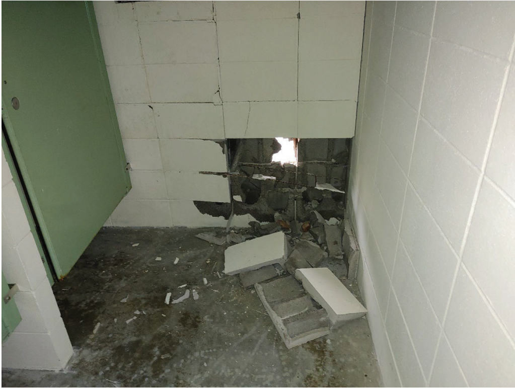
7. The interior view of the impact site.
