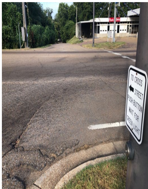
PUSHBUTTONS AND SIGNALS (YET NO CROSSWALKS) Looking West at 5 th Avenue Across 5 th Street
